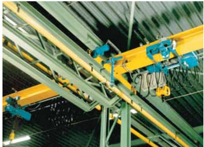
Supply for crane installation
