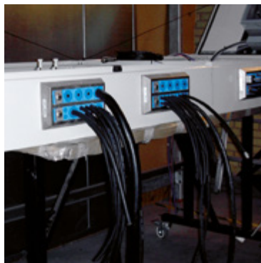
Wind turbine: Roxtec transits for potential equalization as well as the Roxtec standard system for control cabinets in the nacelle.
